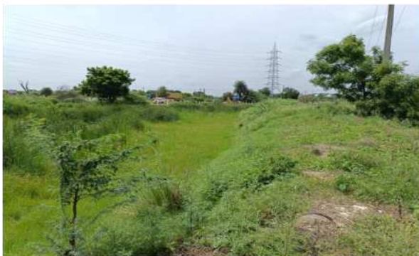
BEFORE EXECUTION Weir No.3 D/S
