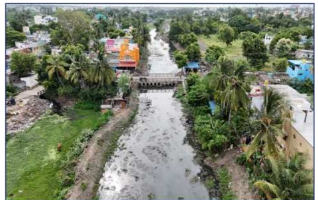
DURING EXECUTION Sadavaram Bridge D/S
