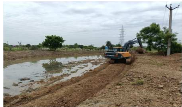
DURING EXECUTION Weir No.3 D/S
