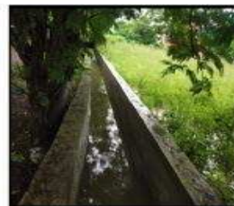
Construction of Rain water Drain in Kamarar Nagar Main Street & Cross Streets in Varadarajapuram Panchayat. 400m Length
