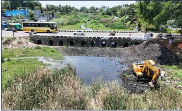
BEFORE EXECUTION Kavalangate Bridge
