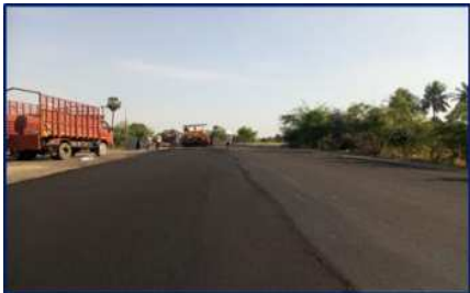
Kanchipuram Bye Pass (West) at Km 1/600 - 4/8 including Bridge Portion at Km 3/0 - 3/2
