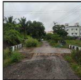
Construction of 2 Nos. of RCC slab culvert of vent 2.00m at Shanthiristannagar at Varadarajapuram Panchayat
