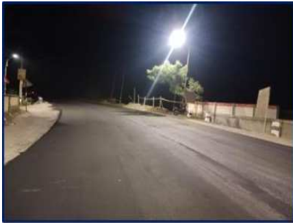
Km 3/650 - 4/150 & 5/050-5/550 of Kanchipuram Wandawasi Road.
