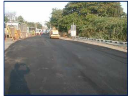
Sadras - Chengalpattu - Kanchipuram - Arakkonam - Thiruttani Road at Km 50/4 - 52/4 & 66/0 - 66/940
