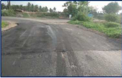
Ullavoor -Thollazhi Road at Km 1/0 - 5/2
