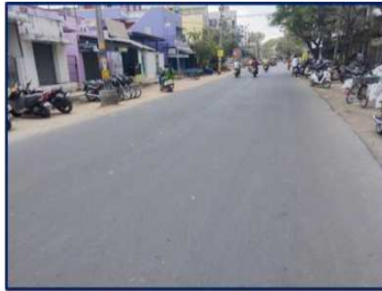
Kanchipuram - Surappan Road at Km 66/8 - 72/2.
