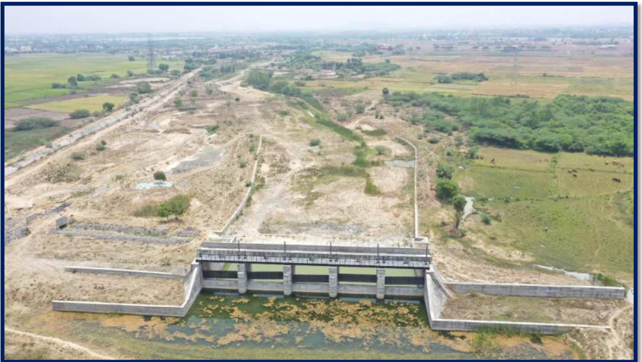
Spillway of Orathur – Arambakkam Reservoir
